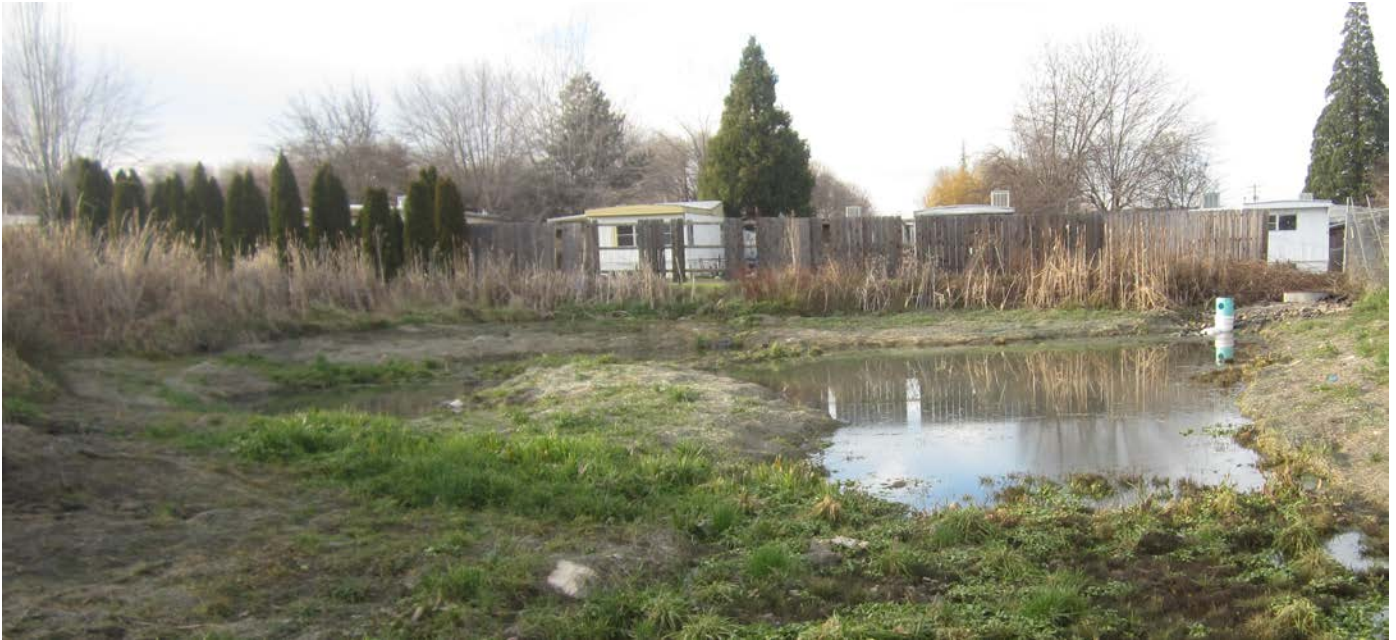
Stormwater wetland in the City of Talent renovated by RVSS to improve stormwater quality and quantity management
